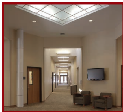
Training center lobby has displacement ventilation.
